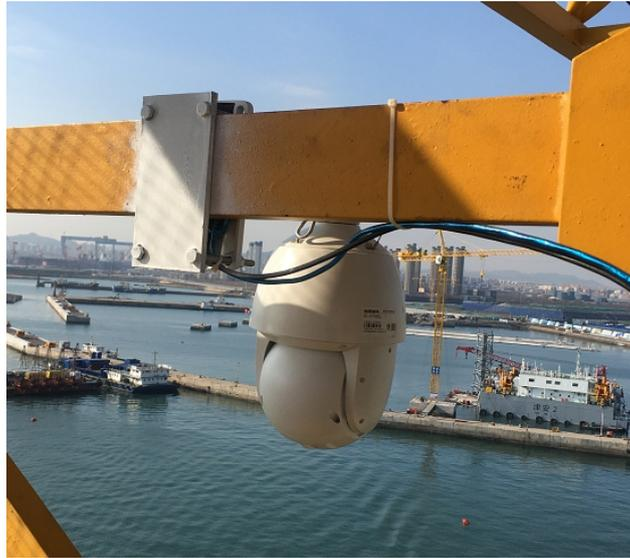
The zoom camera is installed under the trolley or at the root of the main jib on the level-jib tower crane to monitor the lifting state of the hook.
